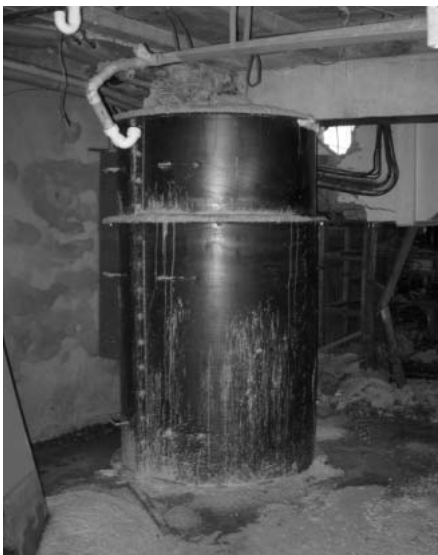
Damaged columns with completed encasement
