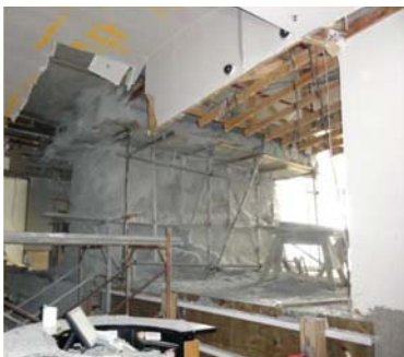
Overall View of Repair Using Shotcrete
