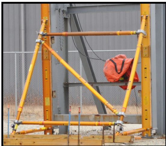
Photo raker using strut
