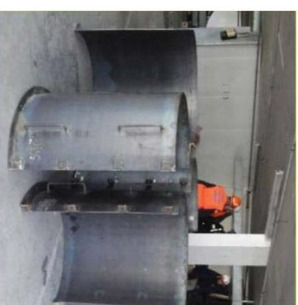
This photo shows a set of half-round steel encasements just prior to erection. Note that the steel encasement is stacked two high in this installation.
