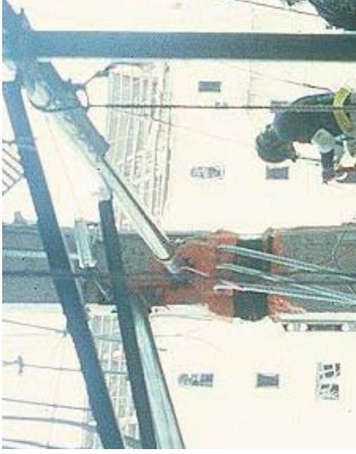
Column F-22 at the Murrah Federal Office Building in Oklahoma City, where the Third Floor used to be. Steel strapping was used as a temporary measure prior to installing a grout filled steel jacket.
