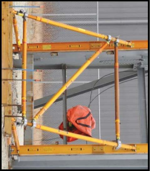
Photo of raker using strut bracing – no wood needed
