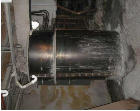
Damaged columns with completed encasement
