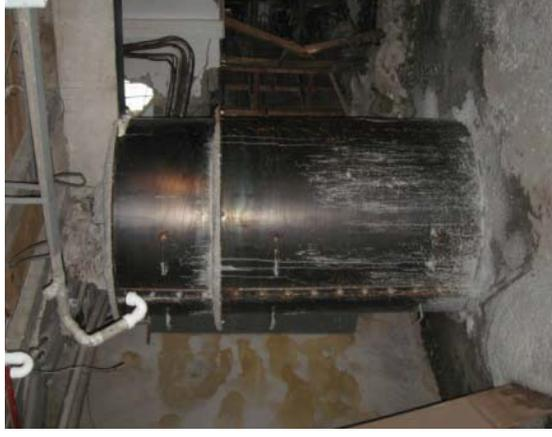
Damaged columns with completed encasement
