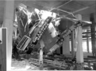
**Each O. rigger was shored Shoring stability failure?**
