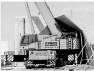
Tilt-up wall braces are vulnerable to buckling (50k, 25ft high wall)
