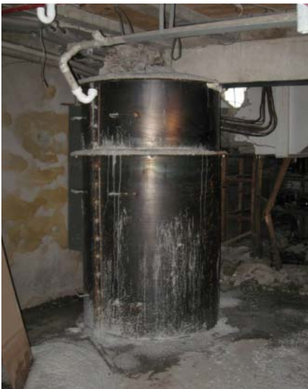
Damaged columns with completed encasement 4-9
