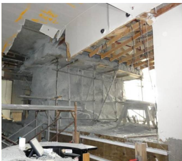
Overall View of Repair Using Shotcrete
