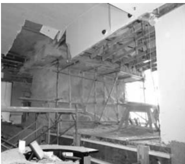
Overall View of Repair Using Shotcrete
