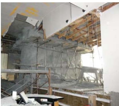
Overall View of Repair Using Shotcrete
