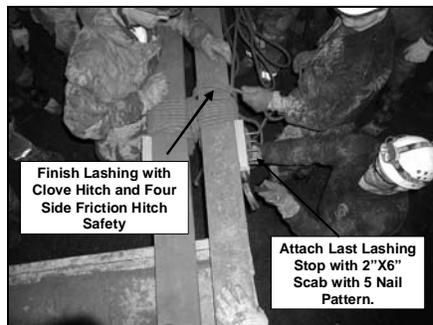
Attach Last Lashing Stop with 2”X6” Scab with 5 Nail Pattern.
