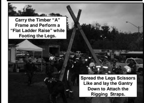
Spread the Legs Scissors Like and lay the Gantry Down to Attach the Rigging Straps.
