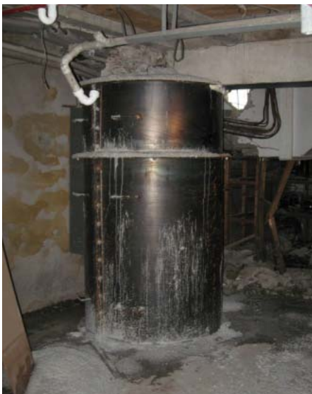
Damaged columns with completed encasement 4-9
