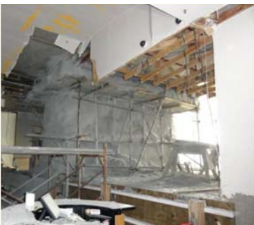
Overall View of Repair Using Shotcrete
