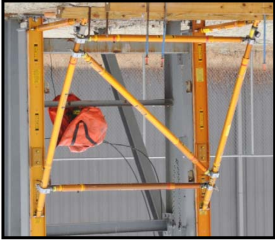
Photo of raker using strut bracing – no wood needed 3-32
