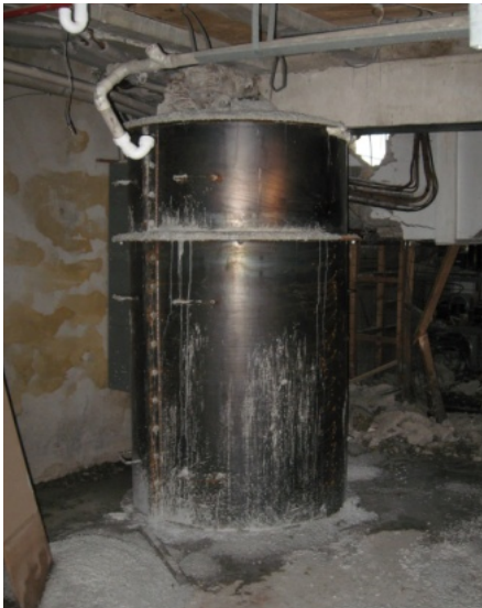
Damaged columns with completed encasement
